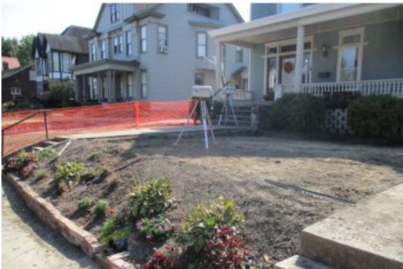
Figure 2: A property after excavation was completed the beginning of October 2020, showing a landscaped area where EPA dug around the plants.
